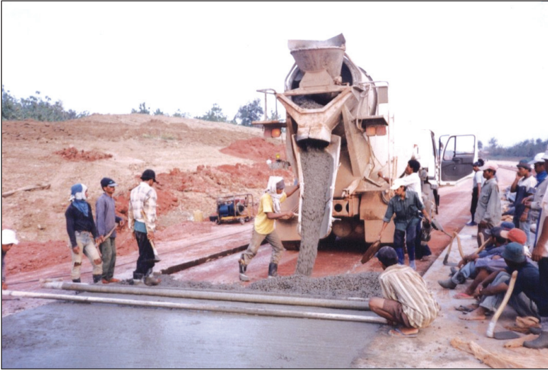
Gambar 41. Tipikal Pengecoran Beton Kurus (Tanpa Subbase )
