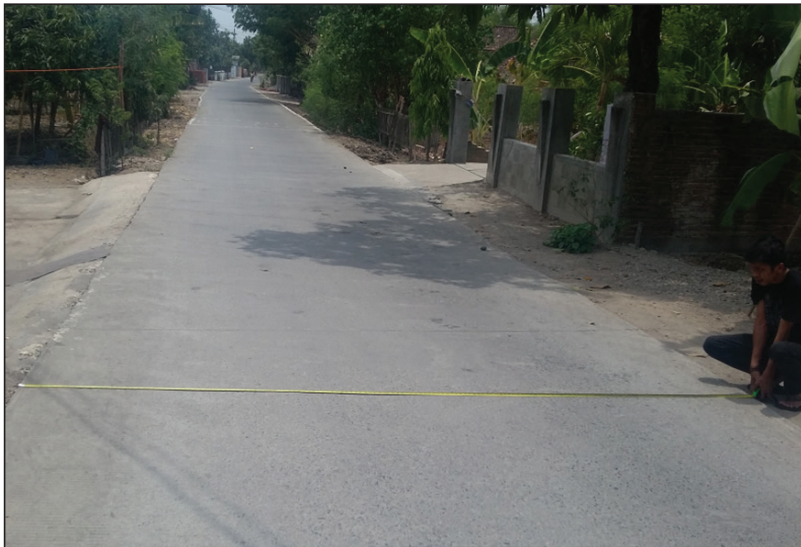
Gambar 12. Tampak Jalan Gulang–Payaman, Tebal Perkerasan Kaku 20 cm (K300), Lebar 4,0 m di Undaan, Kab. Kudus
